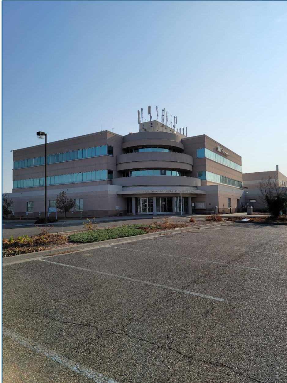
Photograph 2. Exterior Photo - Trios Spaulding Building
