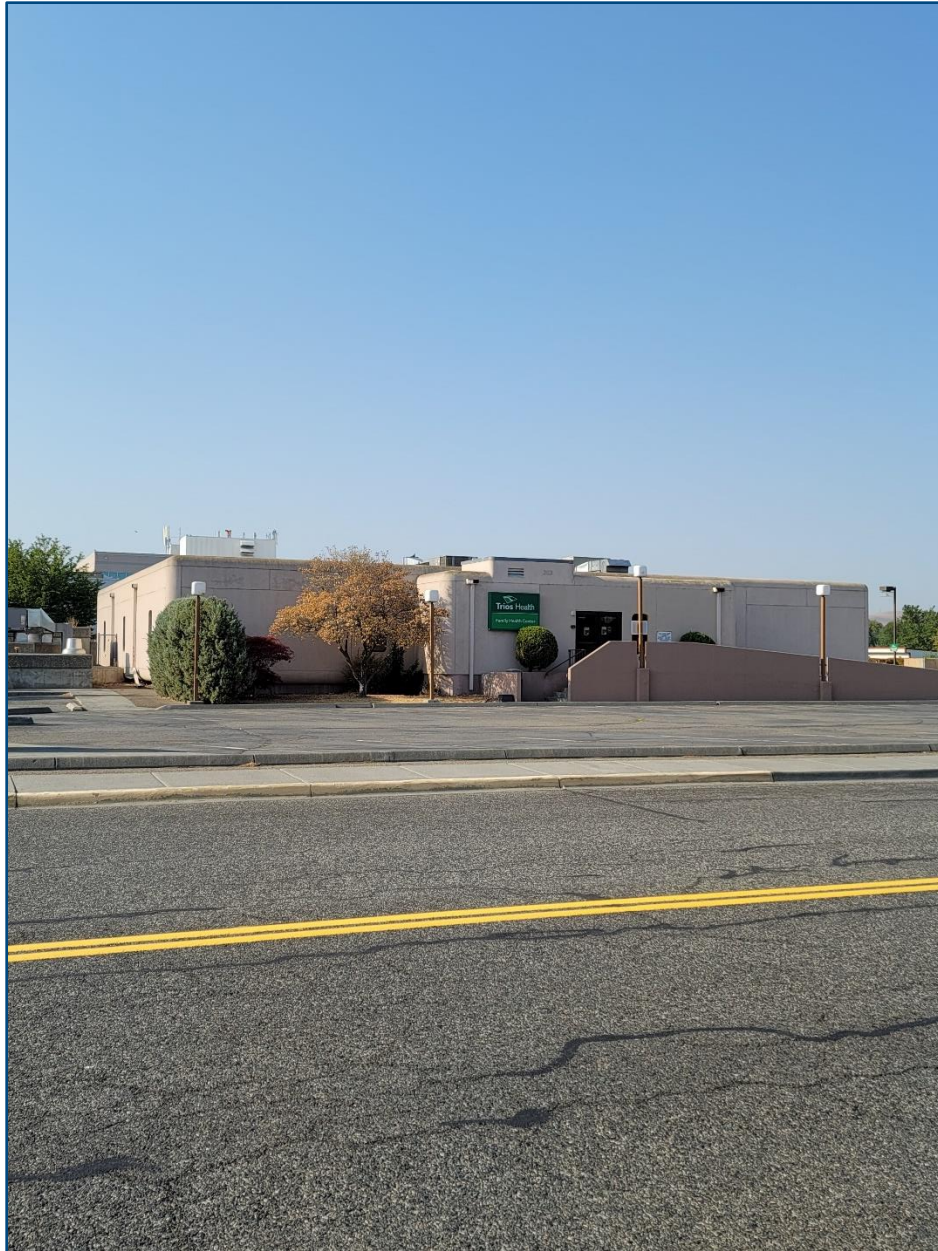
Photograph 3. Exterior Photo - Trios Battelle Building
